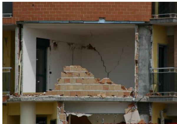
Damaged infilled walls: Emilia Romagna (2012) and L'Aquila (2009)
