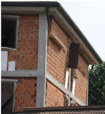
Damaged infilled walls: Emilia Romagna (2012) and L'Aquila (2009)
